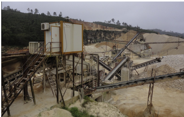
Fig. 2. Primary plus secondary crushing equipment: impact crusher + hammer mill.
