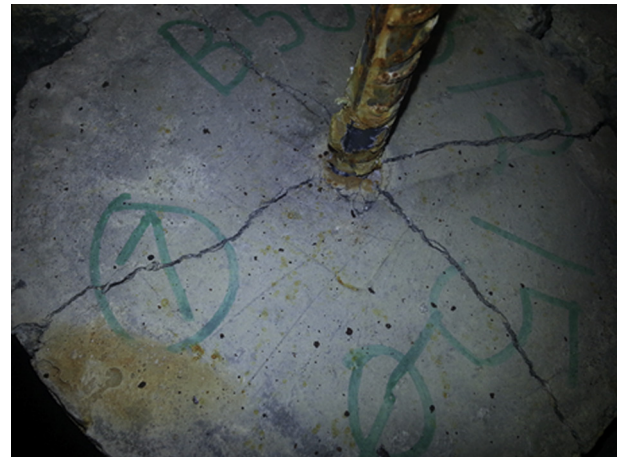
Fig. 4. Cracking at the upper surface of the specimen.
